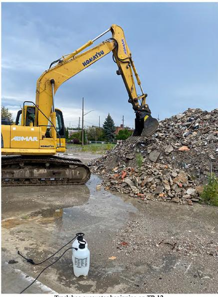
Track hoe excavator beginning on TP-12 (note rainwater which helped minimize dust during excavation)
