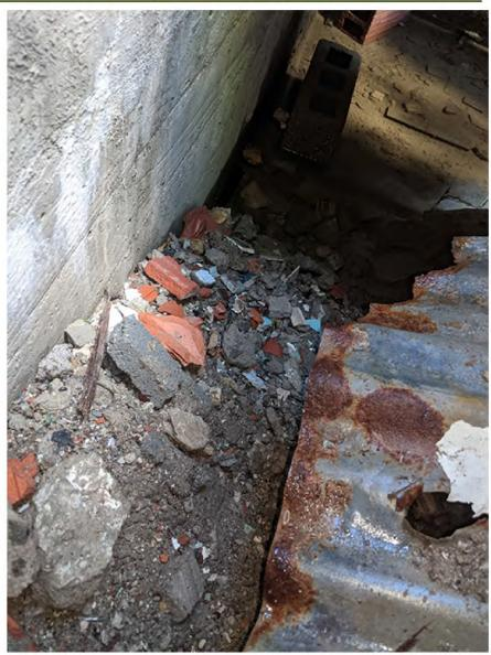
Photo inspection of inaccessible pipe chases under foundation slab with no suspect ACM's observed
