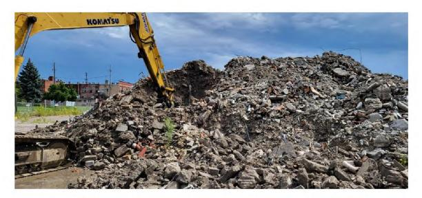
Photo 1: Test pit TP-12-1 (large rubble mound pile south of W. 20th Street) being excavated for sampling.
