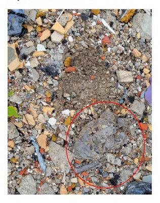
**Photo 6:** Lead sheeting found near TP-4. Lead sample "VL-2" of building debris surrounding sheeting was collected for analysis of total lead and for toxicity characteristic leaching procedure (TCLP) analysis.
