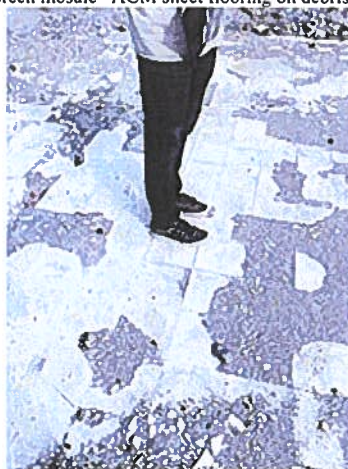
9x9 ACM Floor tile field on the north side of demo site
