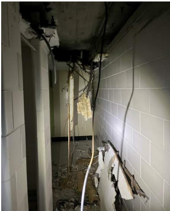
Photo 67: Partially demolished interior fixtures at previously occupied area. Exposed electrical wires and falling debris hazards.
