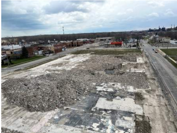
Photo 5: Rubble and debris on site. Open pits, exposed reinforcing, etc. may represent safety hazards.
