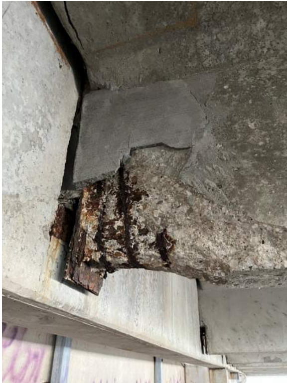
Photo 33: Typical severe spall at joist stem. Exposed corroded reinforcing and embed plate. Spalling of previous repair mortar observed.
