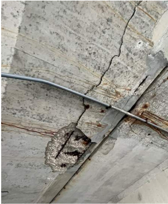
Photo 37: Typical soffit spall at Precast T joint.
