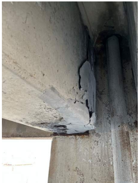
Photo 32: Spall at joist stem bearing at previous repair mortar and corroded bearing plate.
