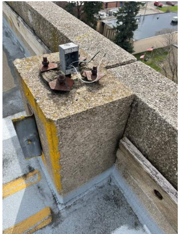
Photo 64: Missing rooftop light fixture with exposed wires.
