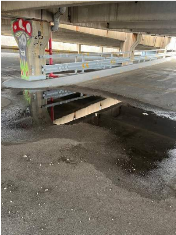
Photo 53: Observed area of ponding below drain above.
