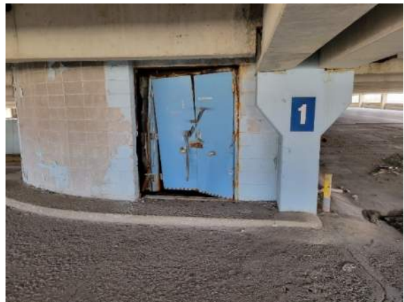
Photo 20: Damaged door at mechanical area at level 1 mechanical room.
