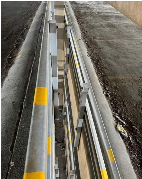
Photo 59: Fall hazard at interior ramps gap between slab sections.
