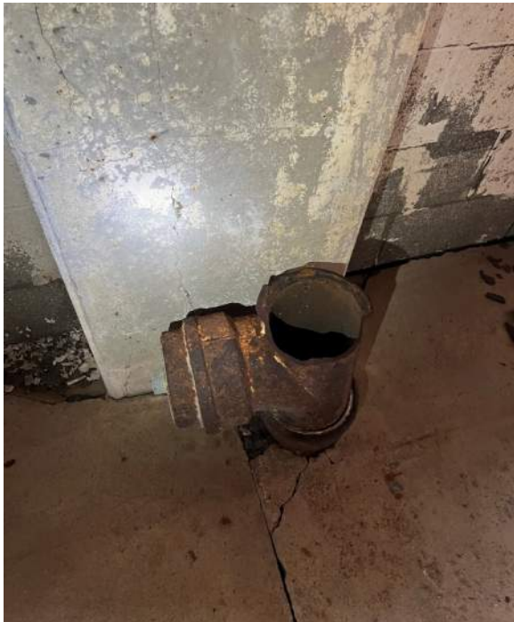
Photo 55: Broken iron drainpipe.
