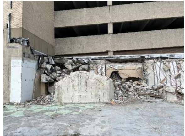
Photo 8: Rubble and debris at partially demolished structure adjacent to parking garage. Falling concrete hazard observed.
