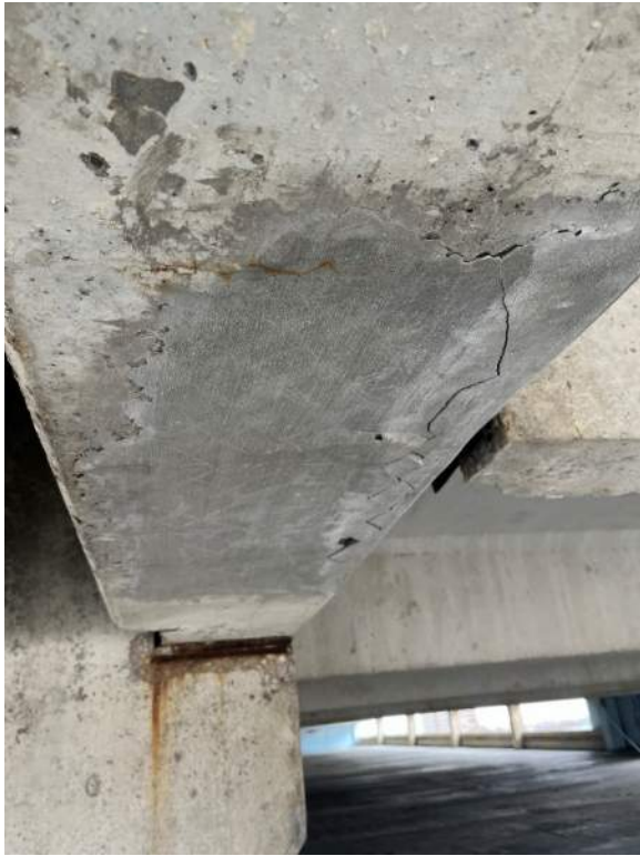
Photo 21: Typical moderate beam spall
