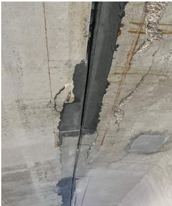
Photo 35: Typical soffit spall at Precast T joint. Spalling of original and repair materials observed.
