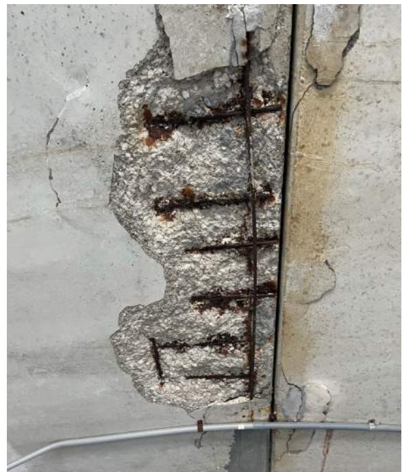
Photo 36: Severe spall of soffit/precast flange. Highly corroded exposed reinforcing.
