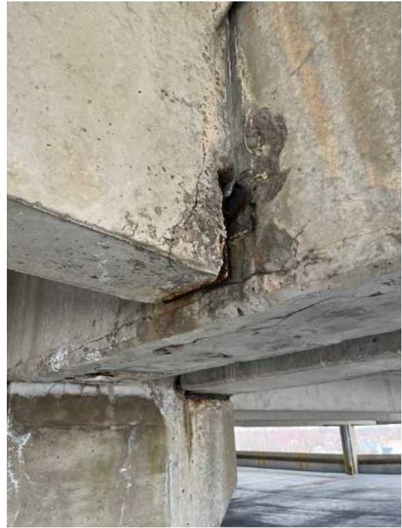
Photo 22: Typical moderate to severe beam spall at joist bearing. Moderate joist stem spall.
