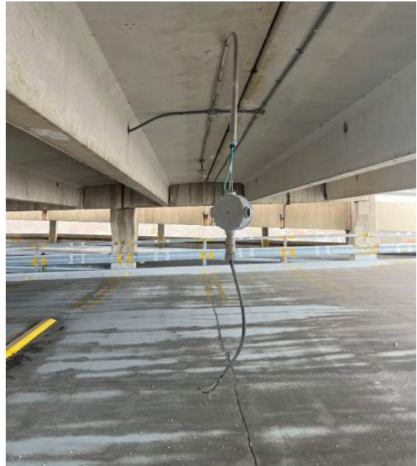
Photo 62: Missing light fixture with detached box and exposed wires.
