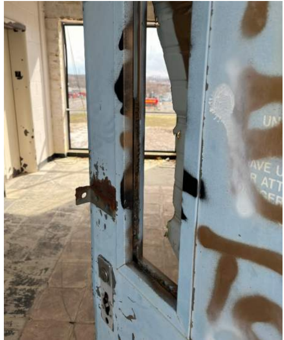
Photo 14: Unsecured elevator lobby door. Weld plate dislodged.
