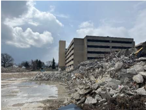
Photo 7: Rubble and debris on site. Exposed reinforcing, falling concrete, etc. may represent safety hazards.
