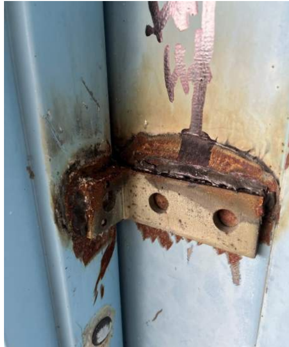
Photo 12: Typical welded shut elevator lobby door (from inside garage).
