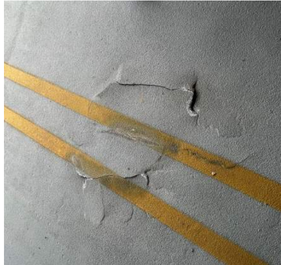
Photo 46: Delaminated epoxy overlay with probable concrete spall below.
