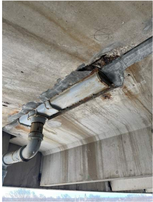
Photo 54: Spalling and deterioration of concrete at trench drain box. Exposed corroded reinforcing and previous repair materials visible.
