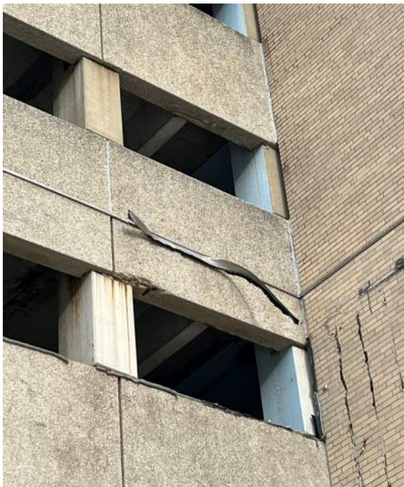
Photo 11: Remaining portion of low roof flashing at east face of garage could fall.
