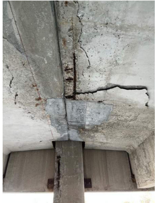
Photo 34: Spall at column and at joist flanges. Spalling of original and repair materials observed. Exposed corroded reinforcing observed.
