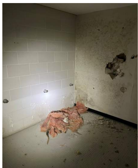
Photo 68: Existing condition of previously occupied area. Mold probable on drywall finished areas.
