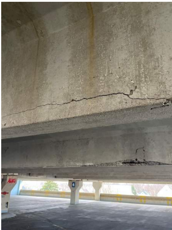
Photo 31: Typical delaminated joist stem.
