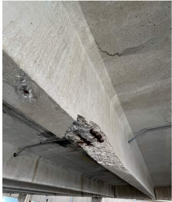
Photo 30: Typical severe spall at joist stem. Exposed corroded reinforcing.
