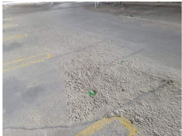
Photo 44: Heavy scaling of top surface of parking deck slab surface. Cracks with failed sealants observed.
