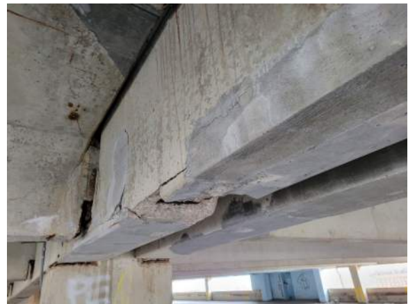
Photo 24: Typical severe beam spall at previous repair.
