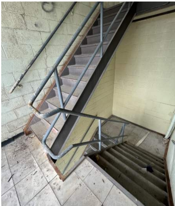
Photo 19: Improper closure of handrail system at stair.
