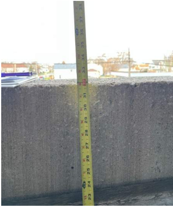
Photo 57: Observed height of perimeter guard walls less than required by code (32" observed, 42" required) for pedestrian fall protection.
