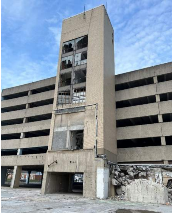
Photo 9: Overall view of east face of elevator/stair tower. Broken window systems do not provide safety closure. Several fall and falling debris hazards exist.
