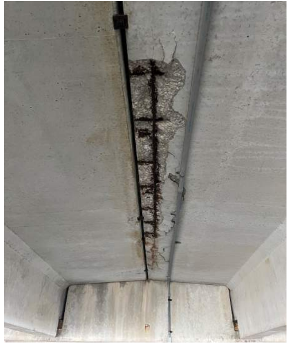
Photo 38: Typical soffit spall at precast T joint.
