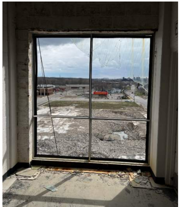
Photo 16: Broken out window system. Fall hazard at accessible area of elevator lobby.
