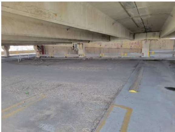
Photo 43: Scaling of top of slab at lower section of garage. Start of newer coated area.
