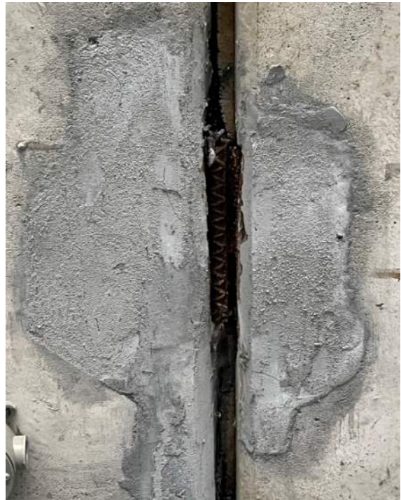
Photo 40: Precast T flange embedded steel connection.
