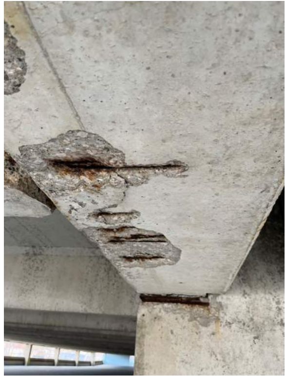
Photo 26: Spalling of beam at stirrups.
