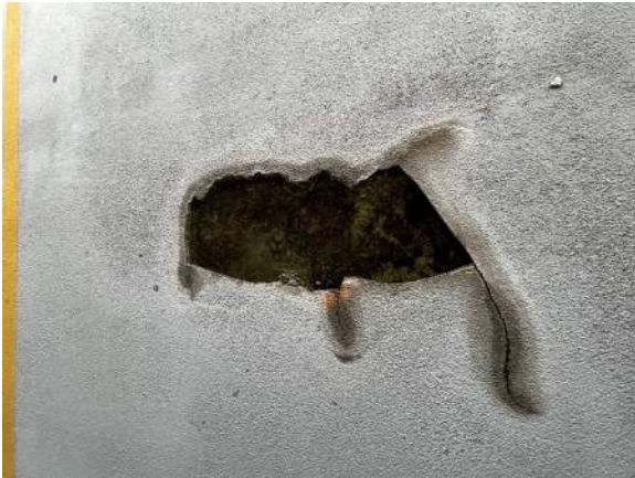
Photo 49: Spall in deck with standing water.
