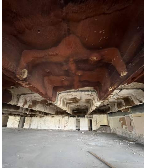
Photo 70: Typical condition of previously occupied area. Water intrusion evident within insulation. Structure above not visible.
