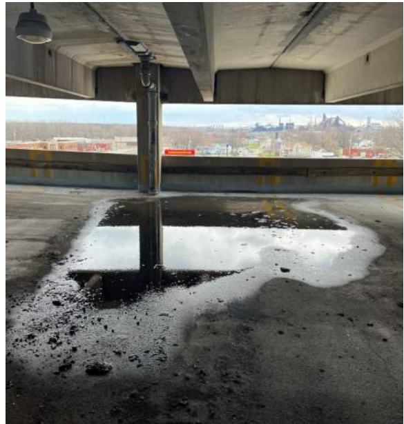
Photo 52: Observed area of ponding below drain above.
