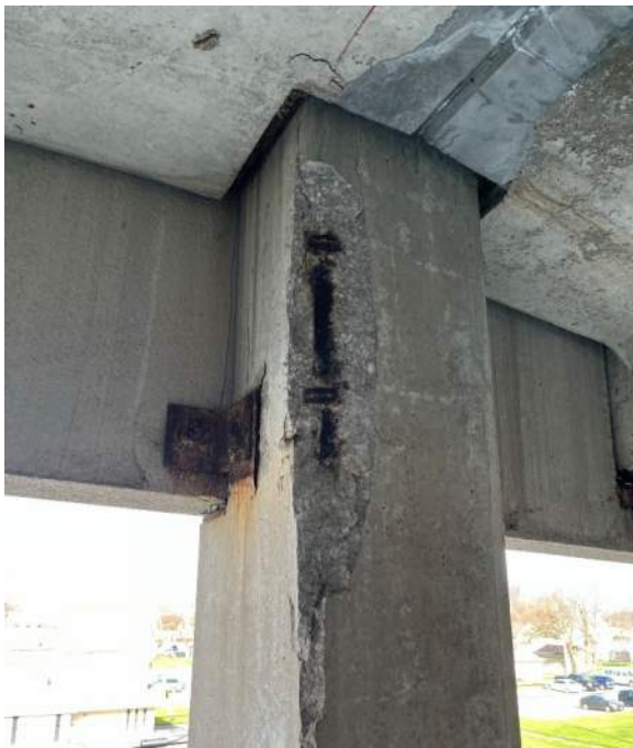
Photo 27: Typical moderate column spall.
