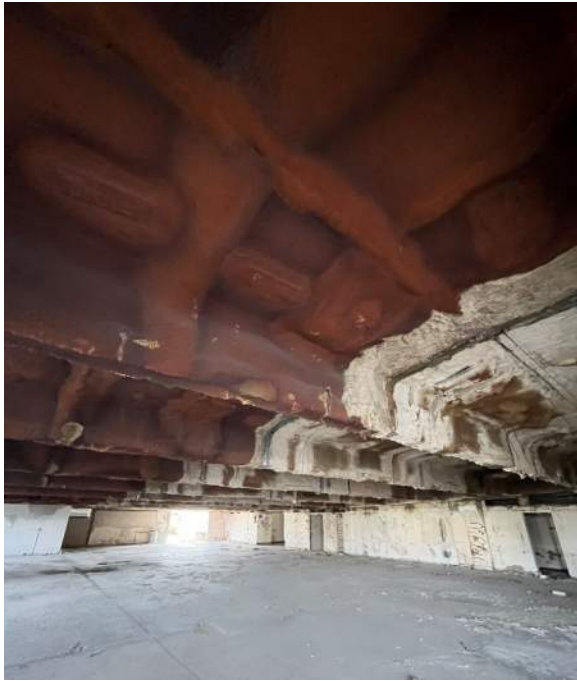
Photo 69: Typical condition of previously occupied area. Water intrusion evident within insulation. Structure above not visible.
