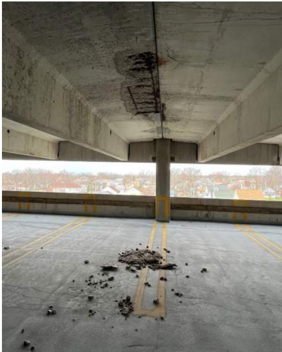
Photo 39: Soffit spall with concrete debris below.
