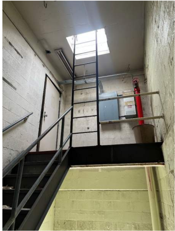
Photo 18: Unsecured roof access hatch at stair tower. Improper closure of hand/guardrail system.
