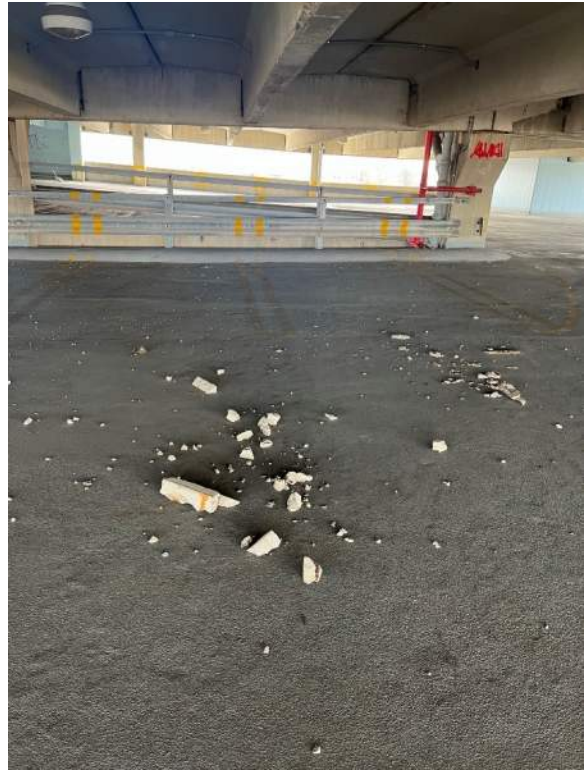
Photo 42: Typical debris on slab at overhead spalls.
