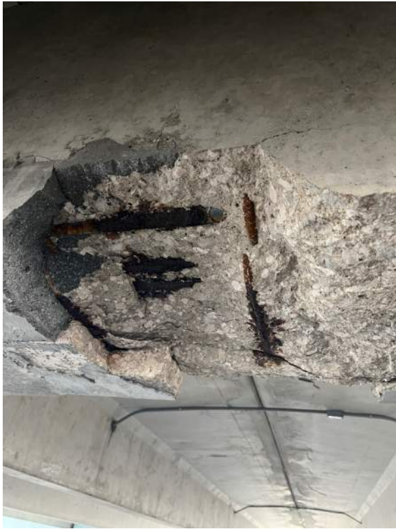
Photo 25: Severe beam spall with exposed corroded reinforcing. spalling of previous repair observed.
