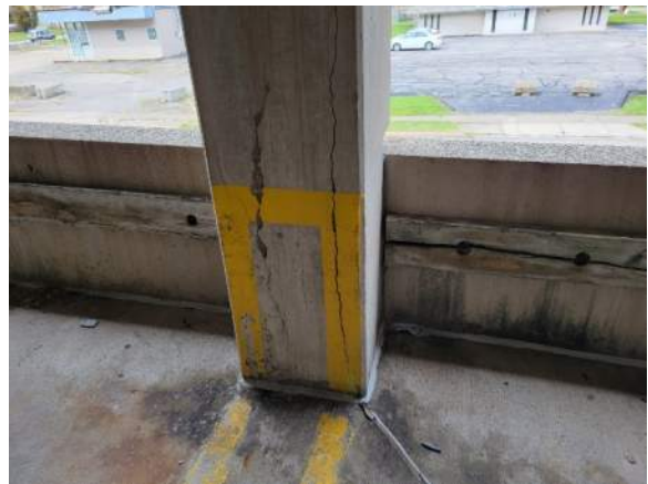
Photo 28: Typical minor to moderate column spall.
