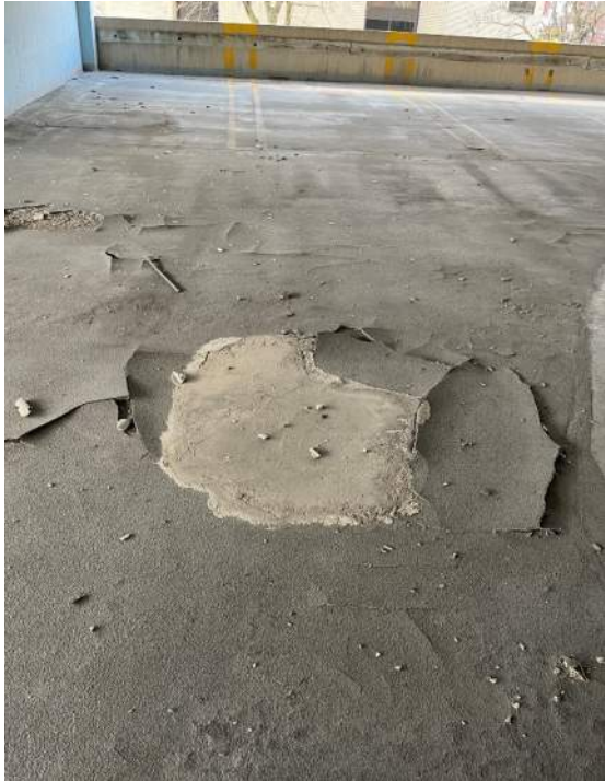
Photo 47: Delaminated epoxy overlay coating.
