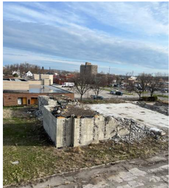
Photo 4: Partially demolished hospital structure on the north side of the site. Exposed portions of embedded rebar and concrete falling hazards exist.
