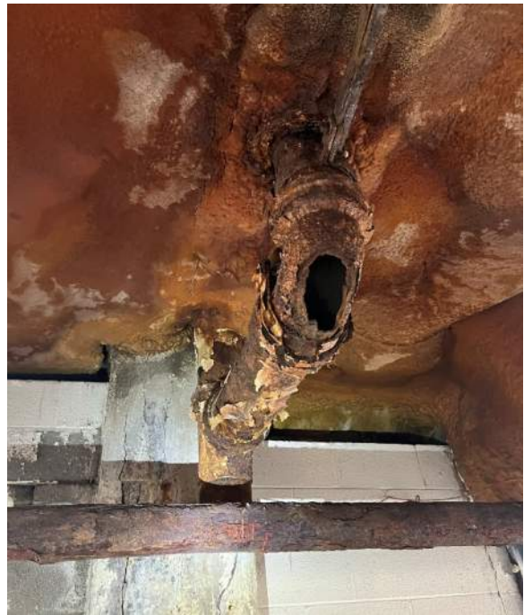
Photo 56: Corroded through drainpipe with missing vertical section at occupied area.
