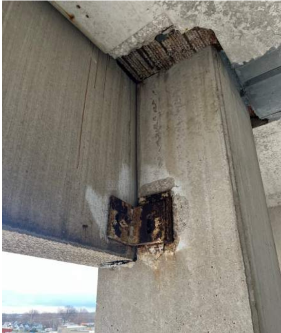
Photo 29: Minor columns spall at corroded precast beam anchor.
