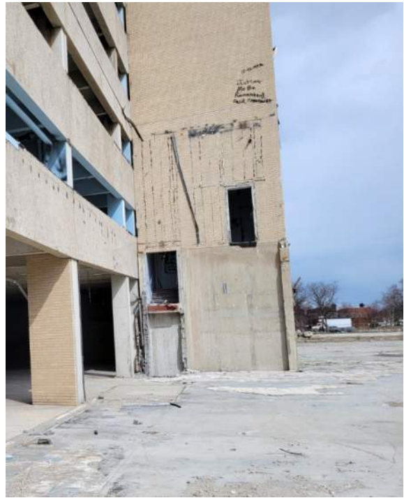
Photo 10: South face of stair tower has two unsecured openings a previous entry to the demolished hospital. Dislodged low roof flashing exists.
