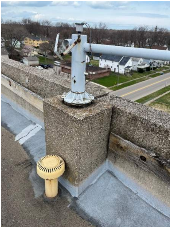
Photo 63: Damaged rooftop light fixture with exposed wires.
