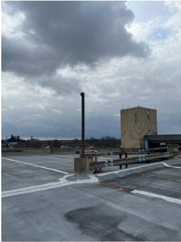
Photo 65: Missing light on post at top level.
