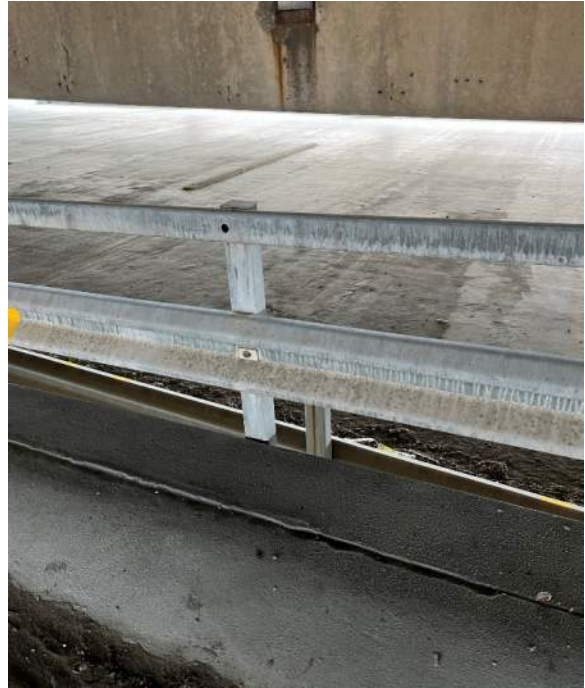
Photo 58: Improper closure at interior ramp vehicular guard rails. Fall Hazard.
