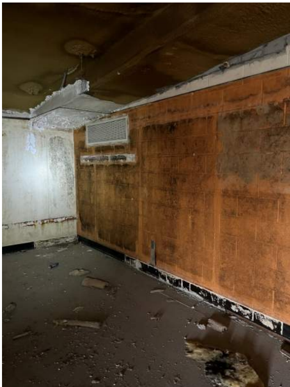
Photo 71: Typical condition of previously occupied area. Mold probable on CMU wall.
