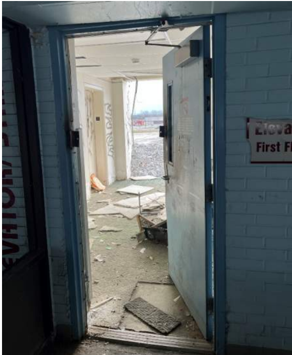
Photo 13: Unsecured Elevator lobby door. Weld plate dislodged.
