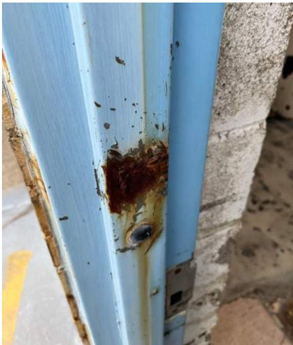
Photo 15: Detached weld plate at door jamb.
