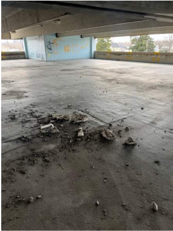
Photo 41: Typical debris on slab at overhead spalls. Size of falling concrete debris represents safety hazard.
