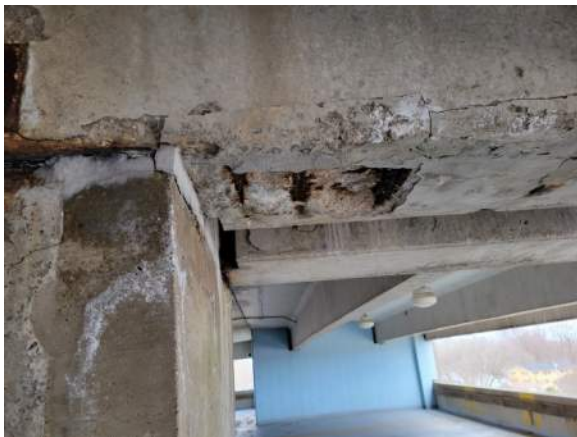
Photo 23: Typical severe beam spall at bearing at column. Efflorescence from de-icing chemicals observed and corroded exposed reinforcing steel.
