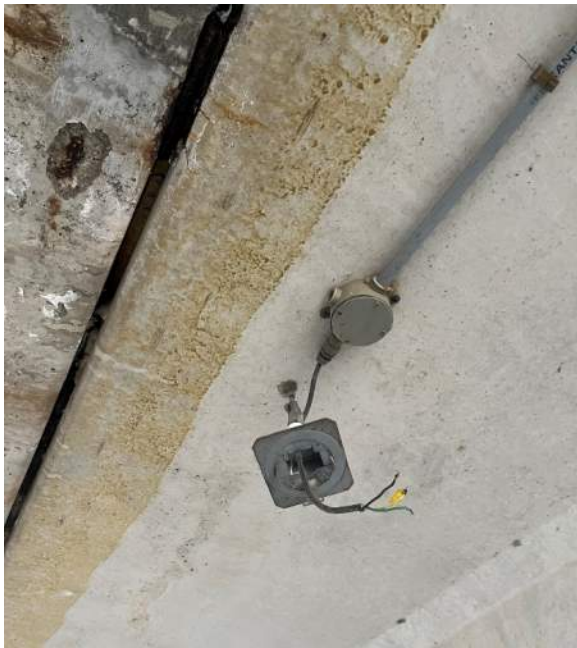
Photo 61: Missing light fixture with exposed wires.
